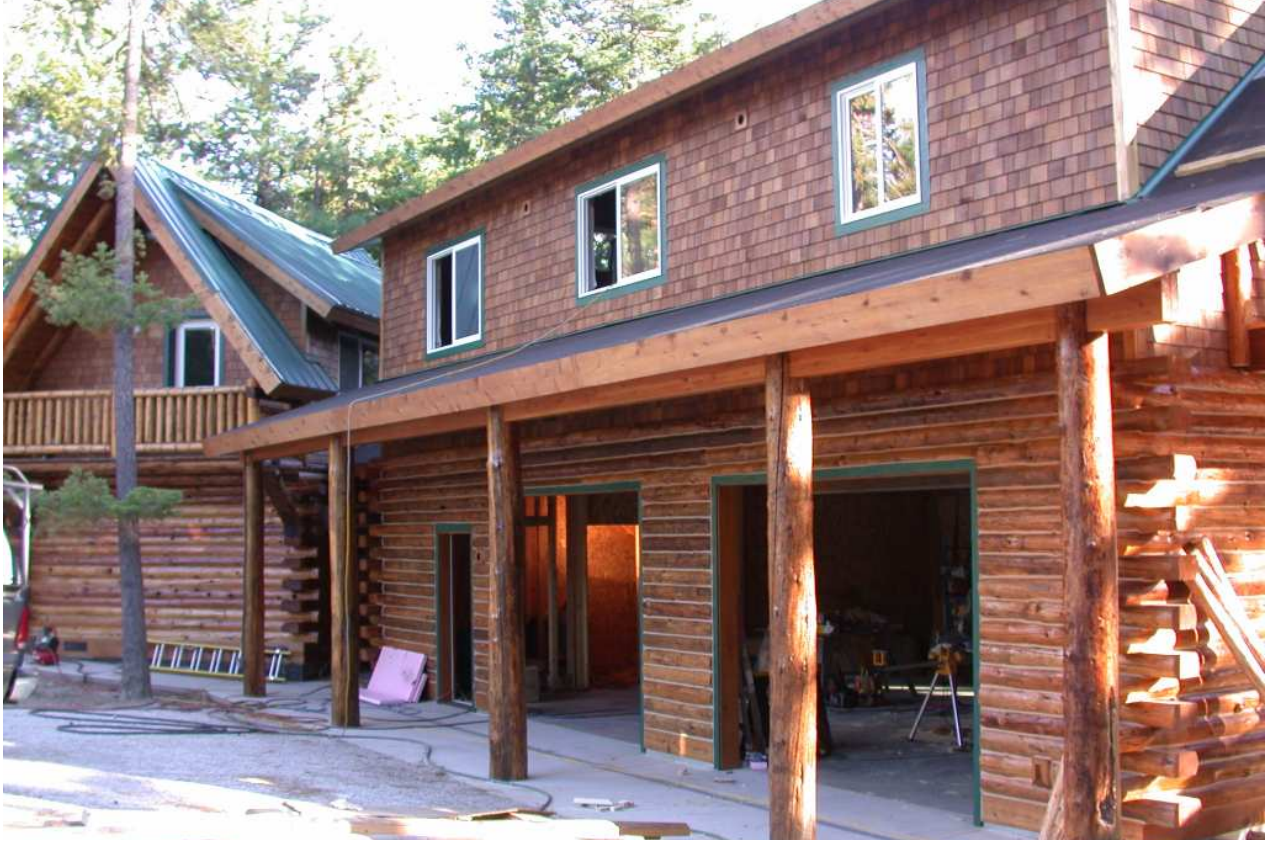
Above: New log siding milled and crafted to closely resemble the adjacent home. Below: New log railings incorporated into existing construction.
