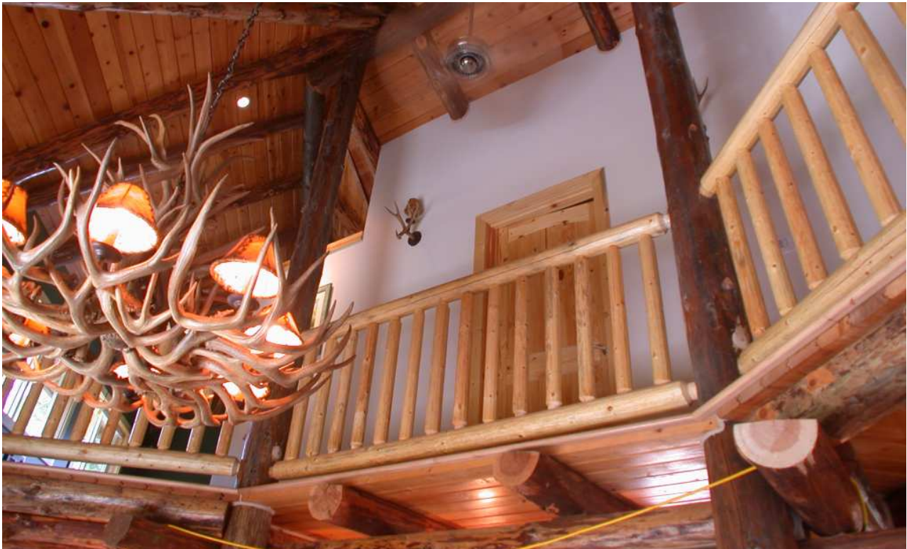
Above: New log siding milled and crafted to closely resemble the adjacent home. Below: New log railings incorporated into existing construction.
