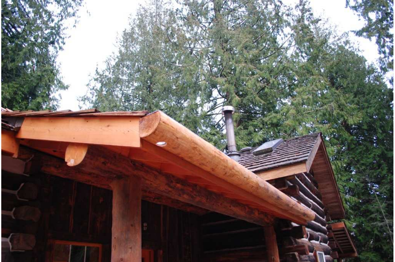
Above: A small diameter log hollowed-out for use with a conventional gutter.
