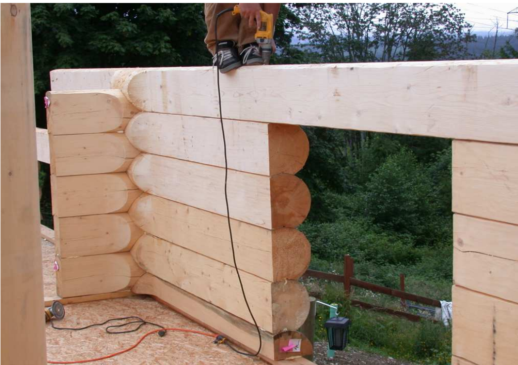
Above: Terry fashioned his own hole saw and jig to bore perfectly sized holes in the uniform round-milled logs.
